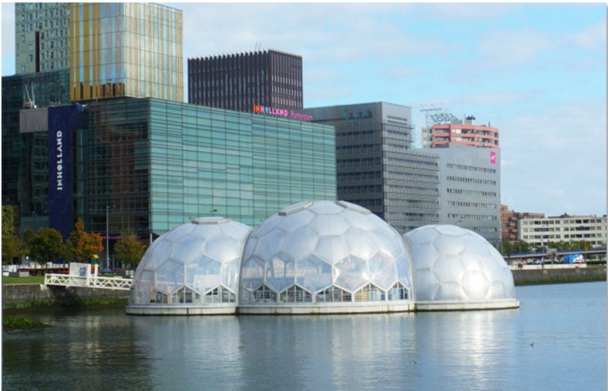
Rotterdam – Floating Pavilion
