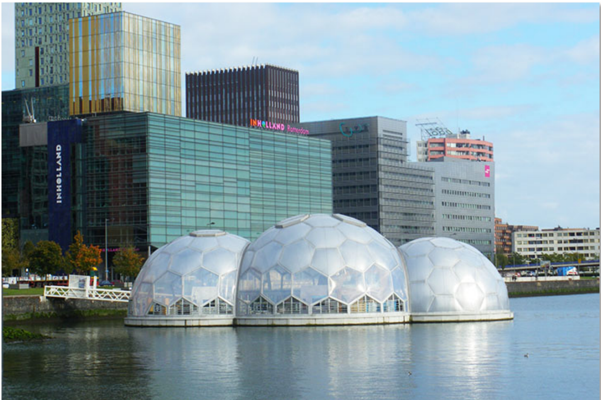
Rotterdam – Floating Pavilion
