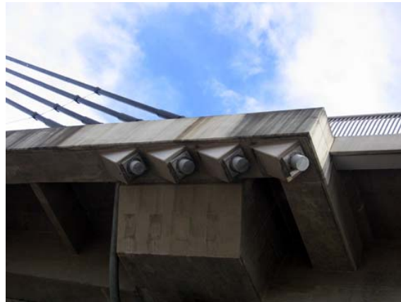
Figure 13: Cable connection
