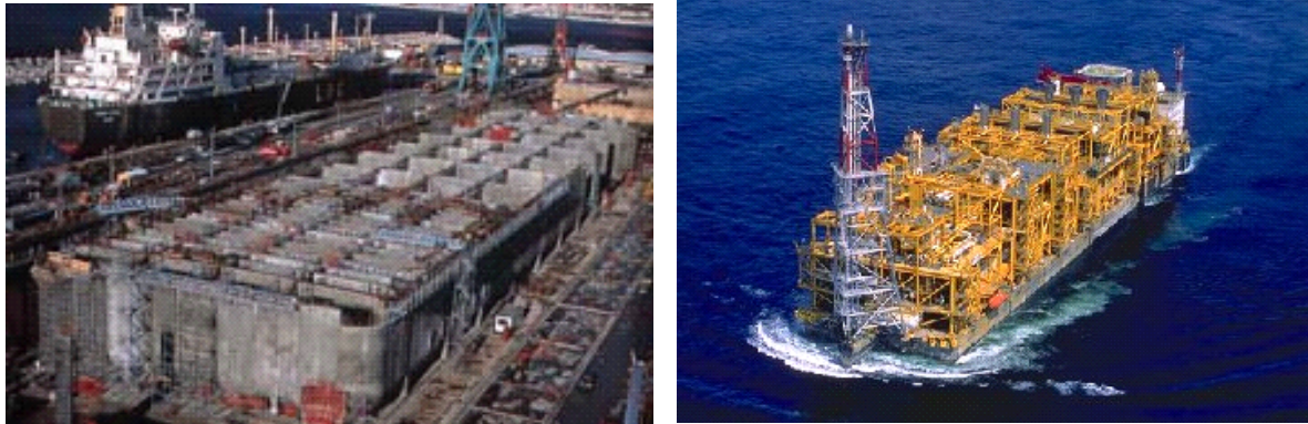
Figure 148: Oil production barge “Nkossa” dam construction and operations (81)
