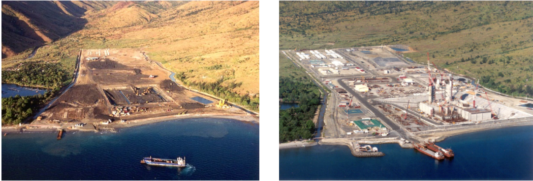
Figure 135: Drydock on the coast of Nigeria to make concrete offshore platforms (83) in construction and operation.
