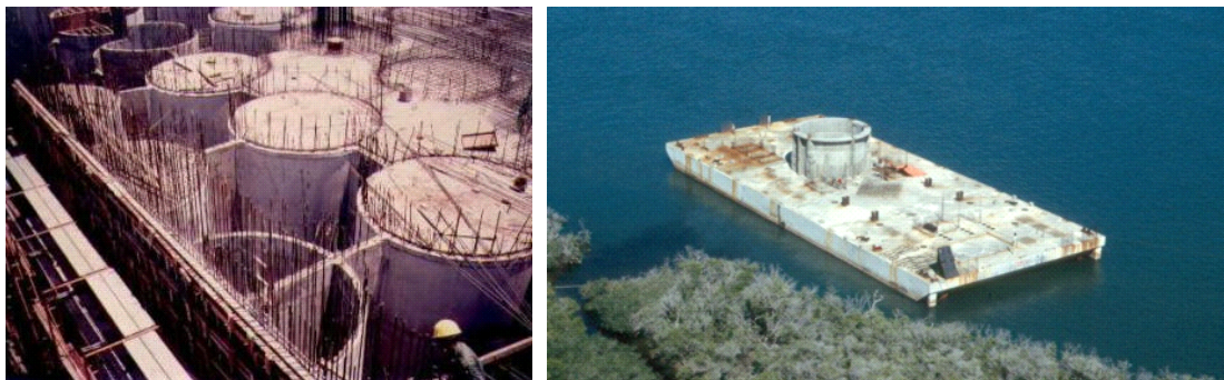
Figure 149: Barge Rofomex I: under construction, Honeycomb system in sight, and afloat (76)
