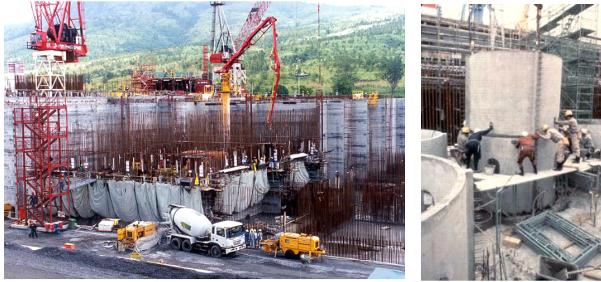
Figure 136: Construction activities typical of a concrete offshore platform (81) (83).
